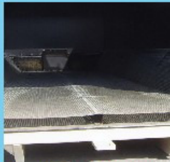
Stainless steel perforated metal to separate liquids from solid waste 3" elevation from floor plan.
